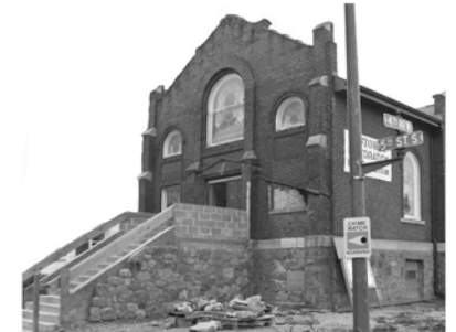
mid-restoration spring of 2010
