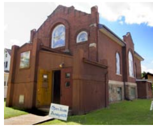
entry annex 1970s
